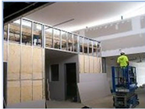
Internal walls in place
